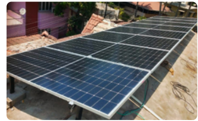
POWERHOUSE PERFORMANCE: PYARELAL FOAMS GOES SOLAR WITH 1 MWP PLANT!
